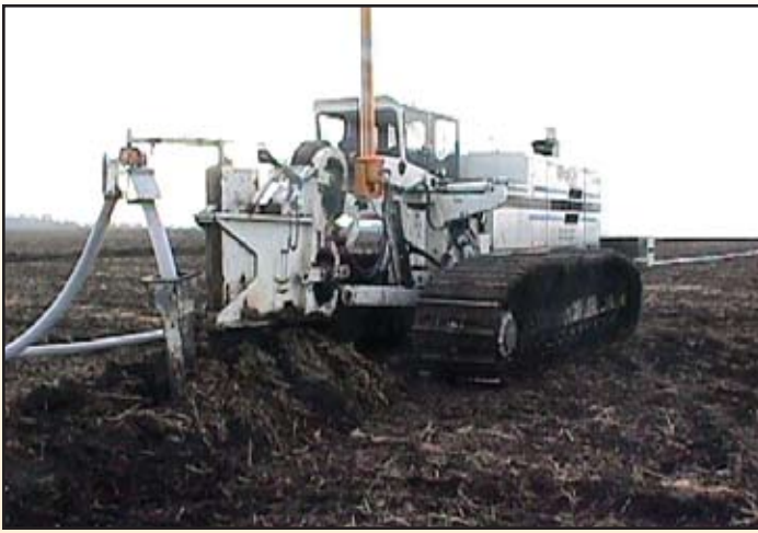
Installing drainage on agricultural land.
